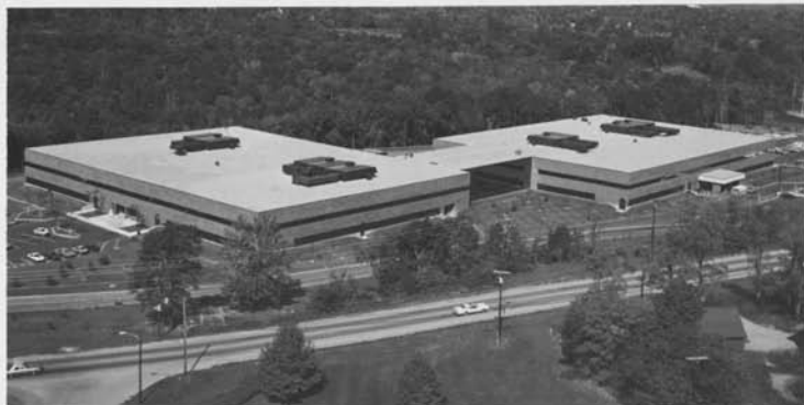
▲ Ground was broken for the Meyers Corners Road buildings in August 1981. From August 6, 1982, to August 16, 1982, one of the largest DP centers
